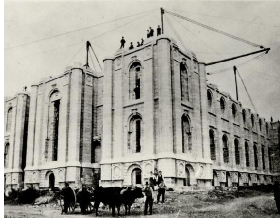
Construction of the Temple 1870 14
